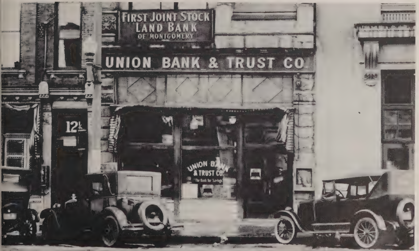
The above building stood next to The First National Bank Building on Commerce until it was demolished in 1962. Picture in 1926.
